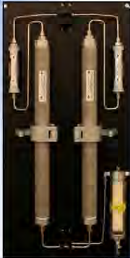
B-3251 H 2 S Scrubber System
